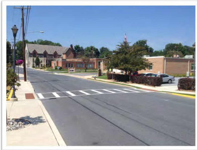
Mid-block crosswalk in Camp Hill
