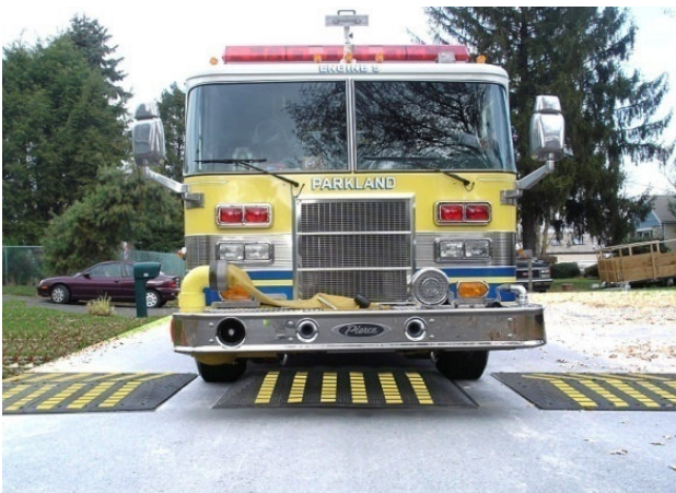
FIGURE 3 - SPEED CUSHION FRONT VIEW
