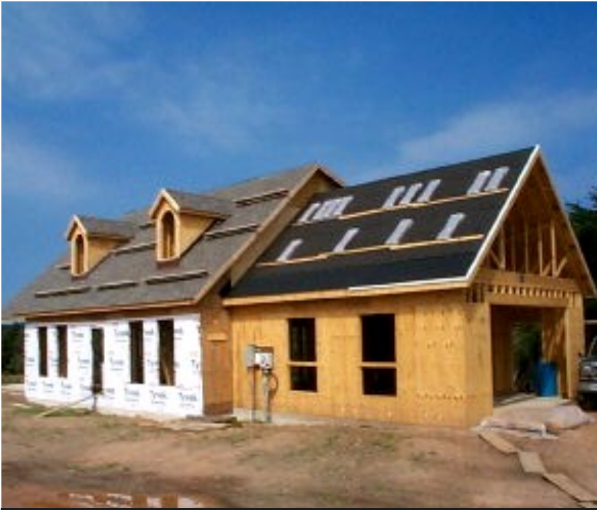
Misc. Residential Construction- Perry County Assessment Office, September, 2000
