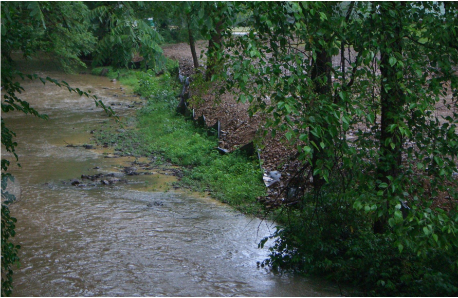
Unattended to Erosion Prevention Measures, June, 2006
