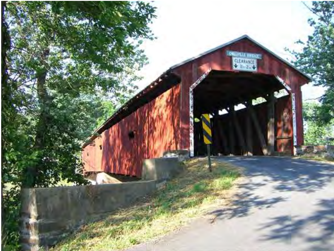
Dellville Bridge before arson fire
