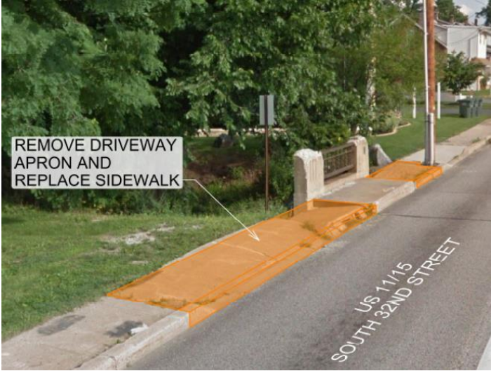
Figure 7 – Proposed sidewalk repairs at 32 nd Street culvert
