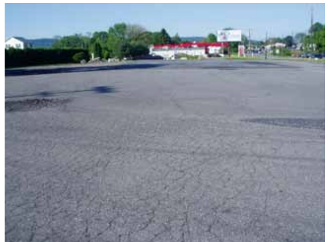
Looking southwest from the eastern edge of the property
