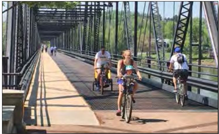
Bicyclists and pedestrians on the Walnut St. Bridge, Harrisburg
