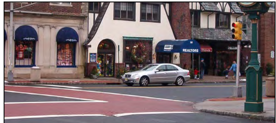
Brick pavers within crosswalks are widely used as traffic calming measures, promoting safer passage for pedestrians.
