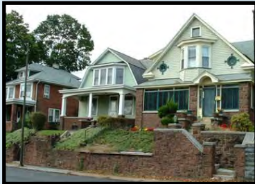
Good-to-Fair: Sound structures that indicate periodic maintenance.
