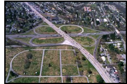
I-83 / Route 22 Interchange
