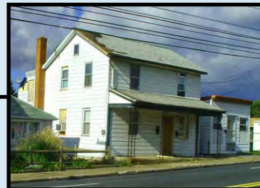
Fair-to-Poor: These are essentially sound structures that have noticeable evidence of erosion along the exterior of the building. Conditions may deteriorate to Poor if remaining unattended for a lengthy period of time. Evidence of Fair-to-Poor conditions includes deteriorated front porches, gutters that are in disrepair, and siding that is no longer intact.
