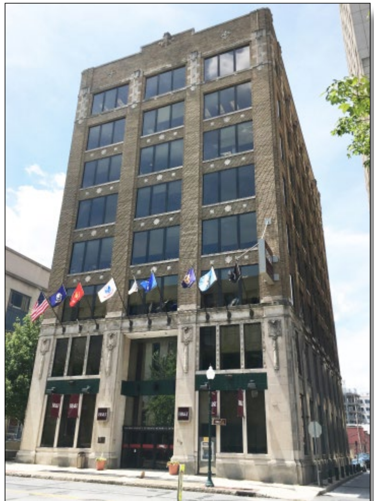
Dauphin County Veterans Memorial Building, Home of Tri-County Regional Planning Commission
