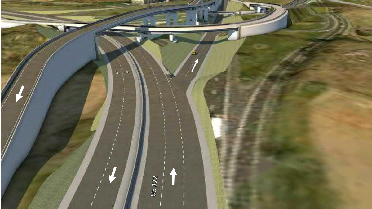
5. Route 422 and Route 322 Exit Ramp
