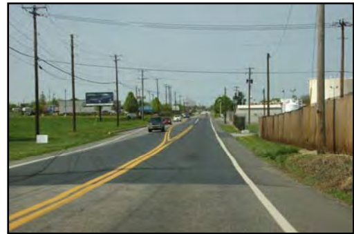
WB Simpson Ferry Road Approaching Sheely Lane/Wesley Drive
