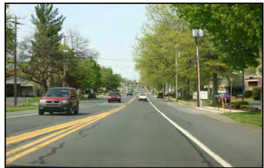
WB Trindle Road – Approaching PA581
