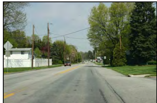
NB St. John's Church Road – North of the PA 581 Overpass
