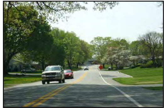
SB Central Boulevard – PA 581 Off-ramp
