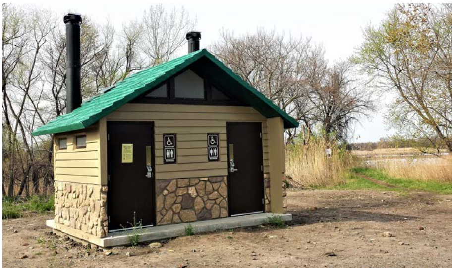
Toilet facilities are very popular at trailheads. This premanufactured pair of composting toilets were successfully installed in an environmentally sensitive natural area.
