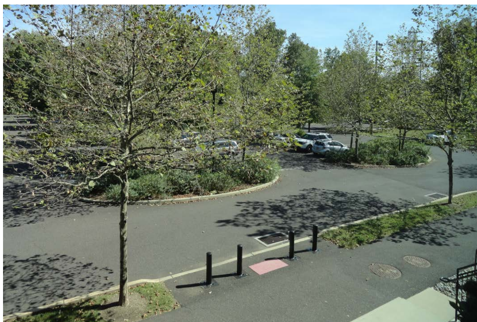
Parking can be pretty. This Trailhead has parking for cars and bicycles along the Schuylkill River Trail in Pottstown PA. . A few years ago it was a treeless, ugly former industrial lot.
