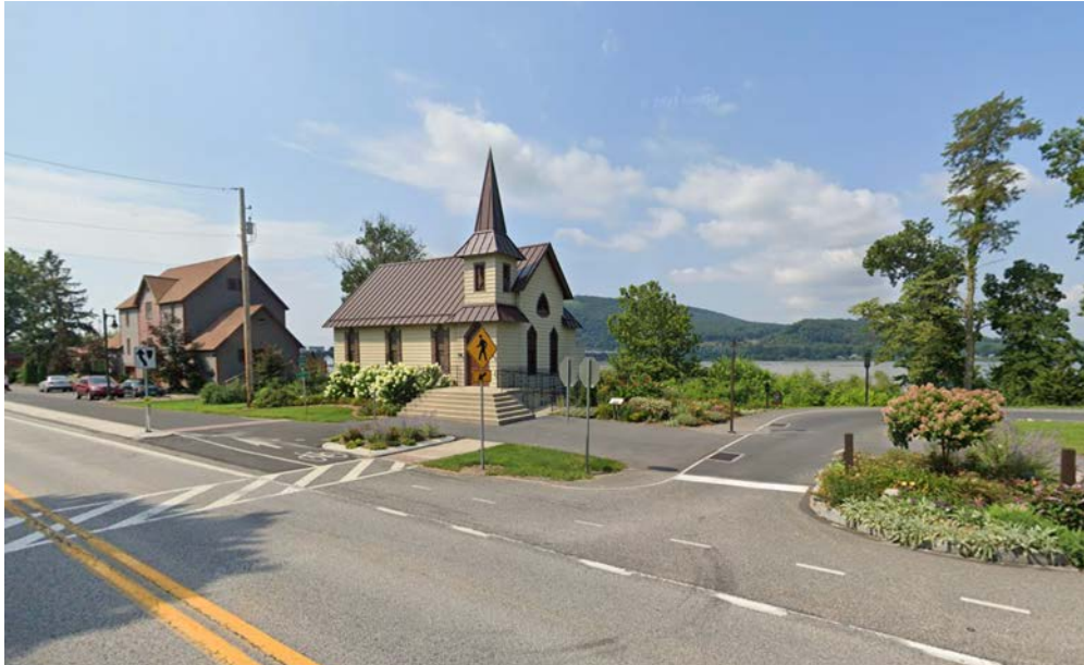
The Fort Hunter Trailhead for the Capital Area Greenbelt in Susquehanna Township provides a model for how well it serves pedestrians and bicyclists
