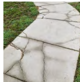
Moderate Cracking
