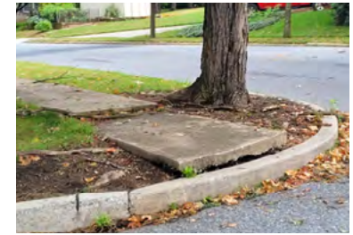
Major Vertical Fault
