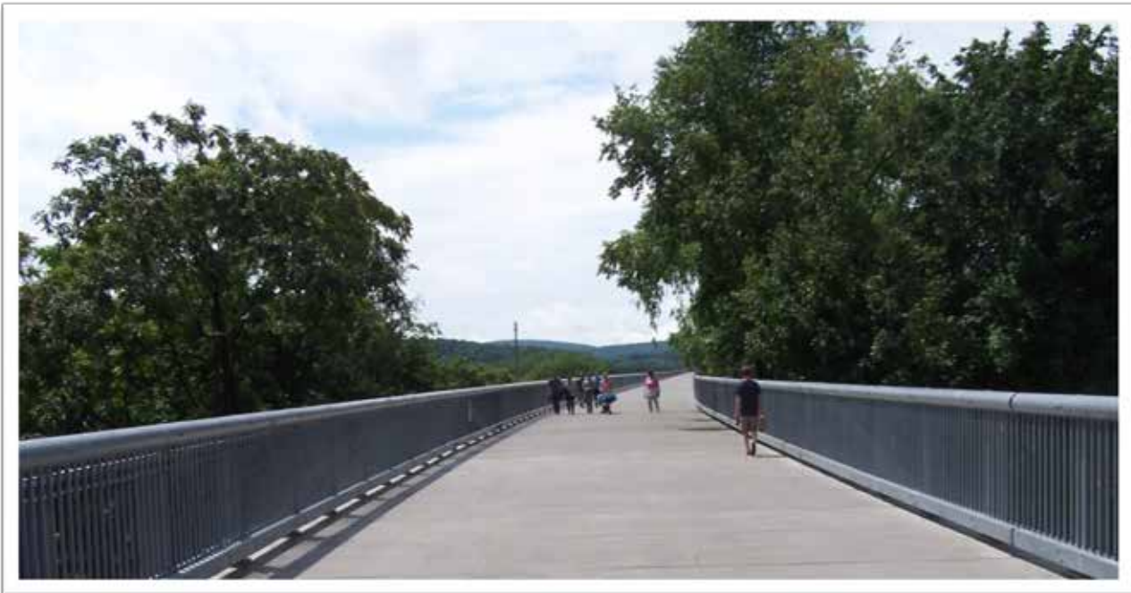
Figure 42: Elevated Park Example – Walkway over the Hudson, Poughkeepsie, NY
