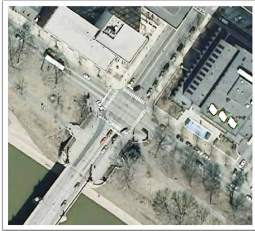
Figure 7: Market Street Bridge and Front Street (Harrisburg)
