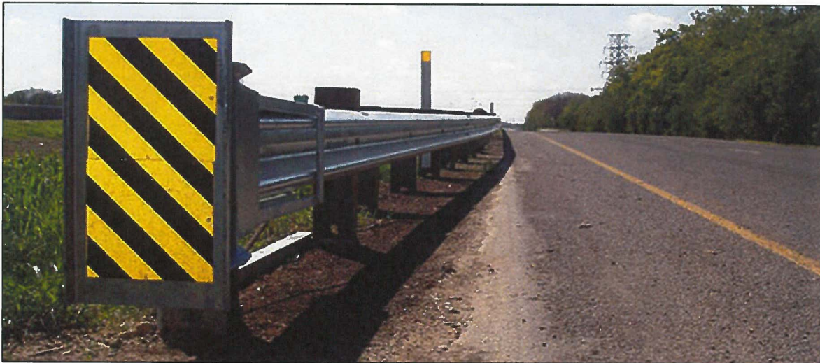
Example of Proper Guiderail End Treatment
