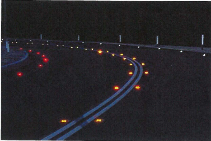
Recessed Reflective Pavement Markings (RRPM)
