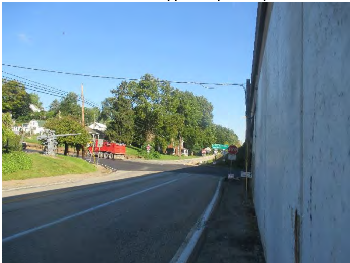
Northbound Approach (Main St)
