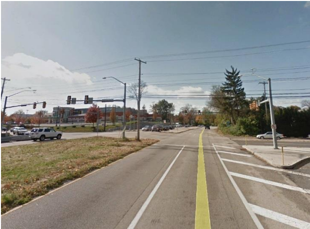
Figure 20 – Camp Hill Bypass southbound, looking south at 21 st Street.
