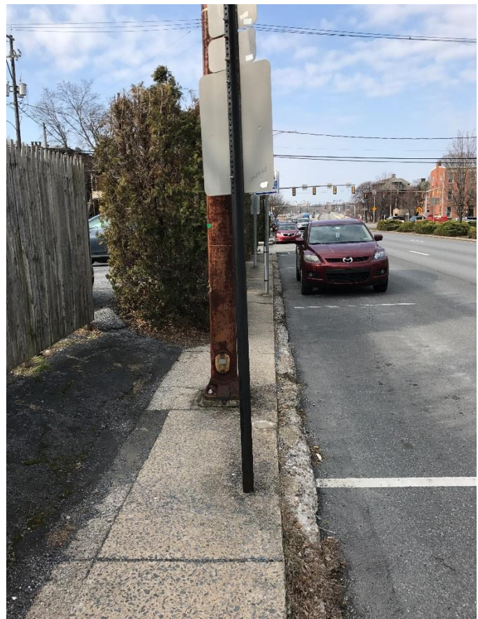
Figure 24 – Sidewalk on Forster Street northbound, looking south. Note poor conditions and numerous obstructions
