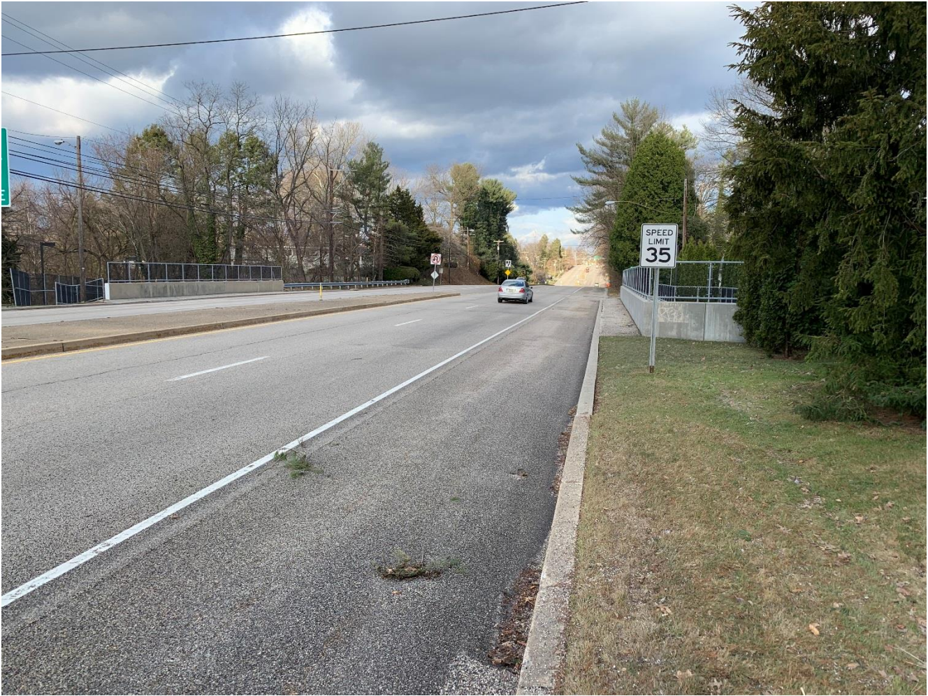
Figure 14 – Cumberland Boulevard pedestrian tunnel, looking north, approaching 27 th Street
