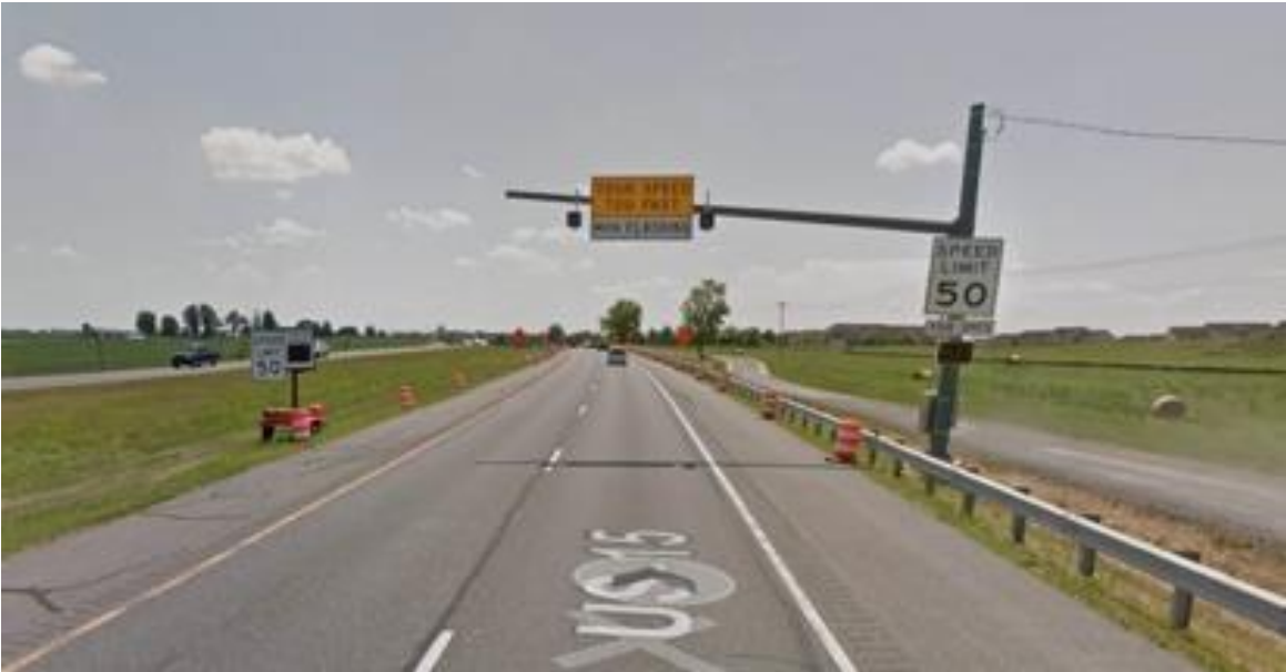
Figure 5 – Example of roadway context transition treatment, US 15 SB, approaching Frederick, Maryland
