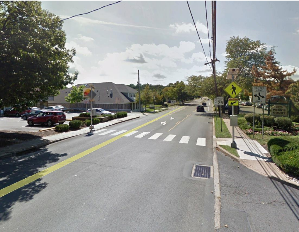
Figure 31 – Rectangular Rapid Flashing Beacon (RRFB), Main Street, Doylestown, Pennsylvania
