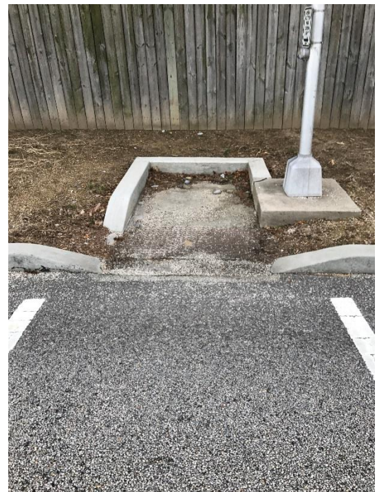
Figure 10 – Existing sidewalk connectivity, 32 nd Street northbound at Brentwater Road
