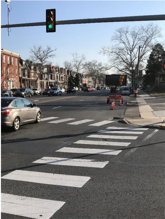
Figure 6 – Continental-style crosswalks, State Street at 13 th Street, Harrisburg
